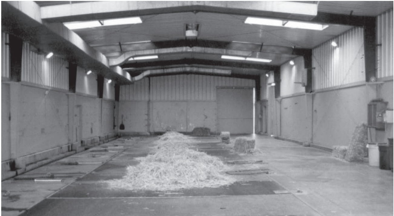
Concrete can act as a heat sink, chilling elephants that lie directly on it. Rubber mats and/or bedding of straw or sawdust can be used to keep the elephants more comfortable.
