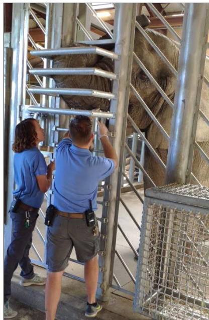
Figure 27 Specially designed mouth and tusk inspection windows, to maintain functional and safe health check procedures in high risk situations ©Martin Kristen.
