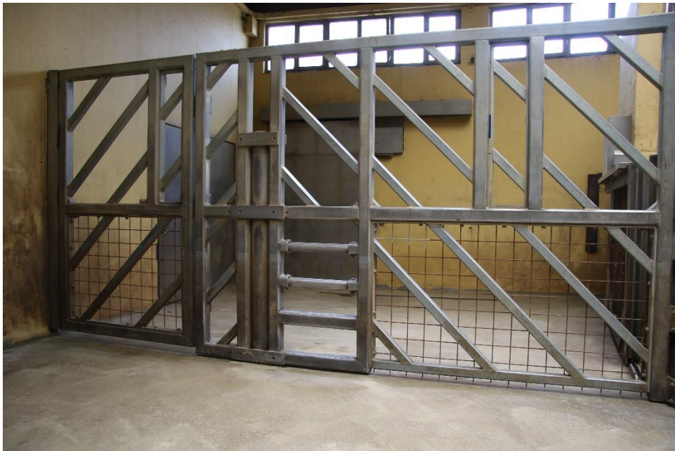
Figure 25 Diagonal bars radiating from centre of the PC wall ©Pavel Vlček
