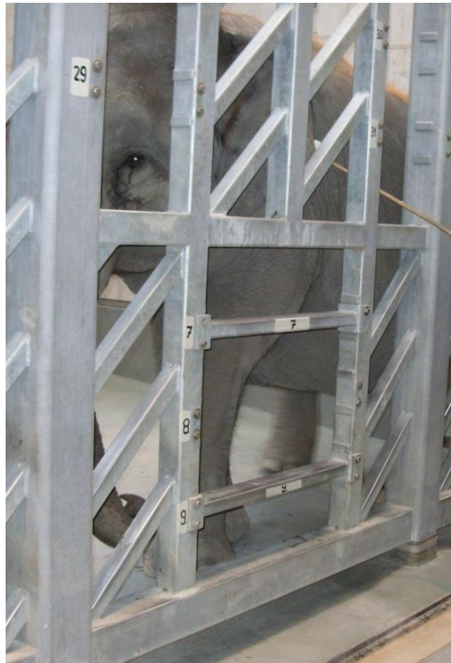
Figure 35 Foot care opening in the training wall in a protected contact system. Note the adaptable crossbars.
